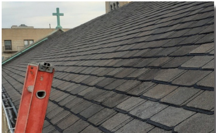
St. John's roofing project.
