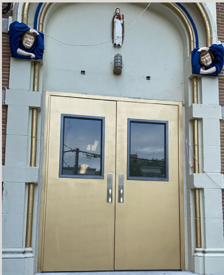
St. Thomas Aquina's new door installation.
